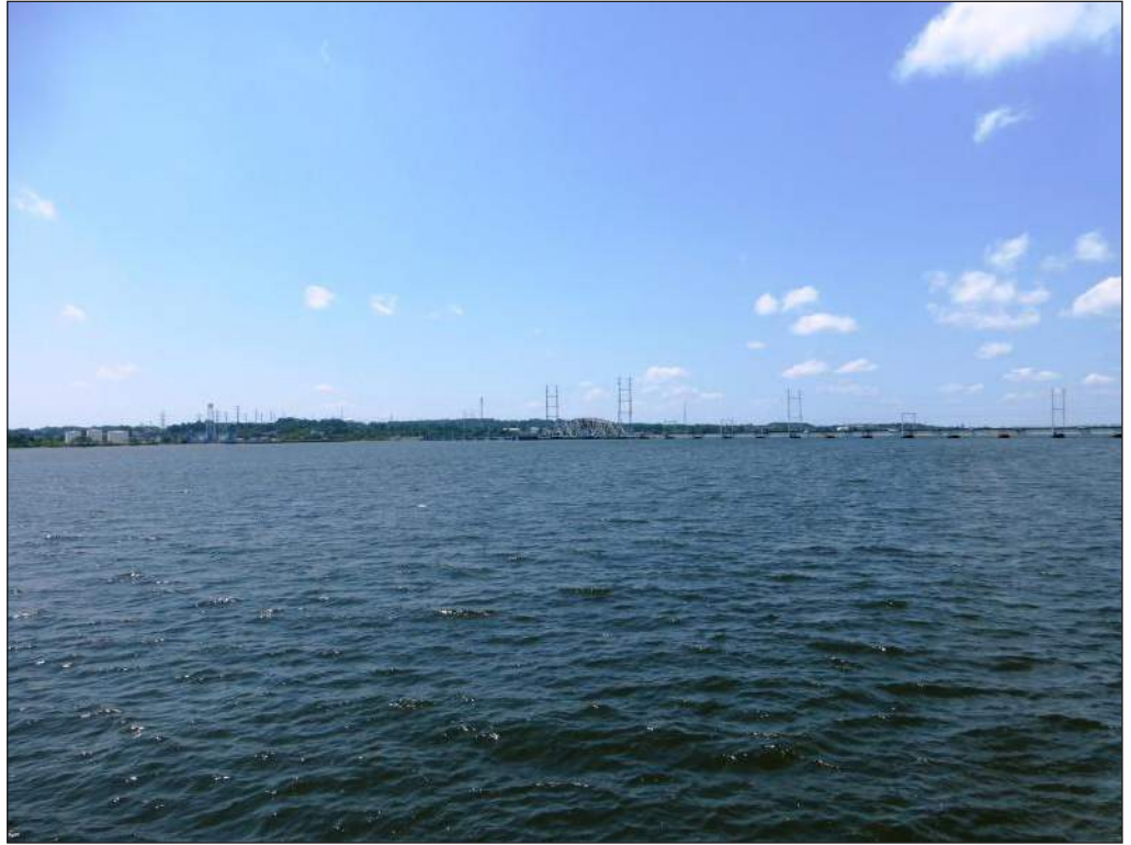
The Raritan River Drawbridge, as seen from the Sadowski Parkway Waterfront Park, looking west. Industrial sites are visible to the southeast but beyond the bridge to the southwest, only trees are visible 1
