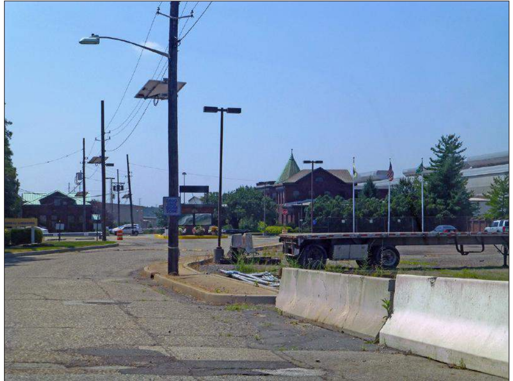
View south from Elm Street at the Gerdau Ameristeel site 3
