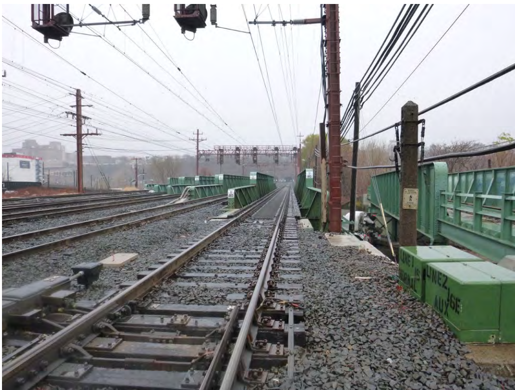
Plate 4.12: View from within the Old Main DL&WRR Historic District toward Palisades, with the Old and New Bergen Tunnels in the background, City of Hoboken and Jersey City.
