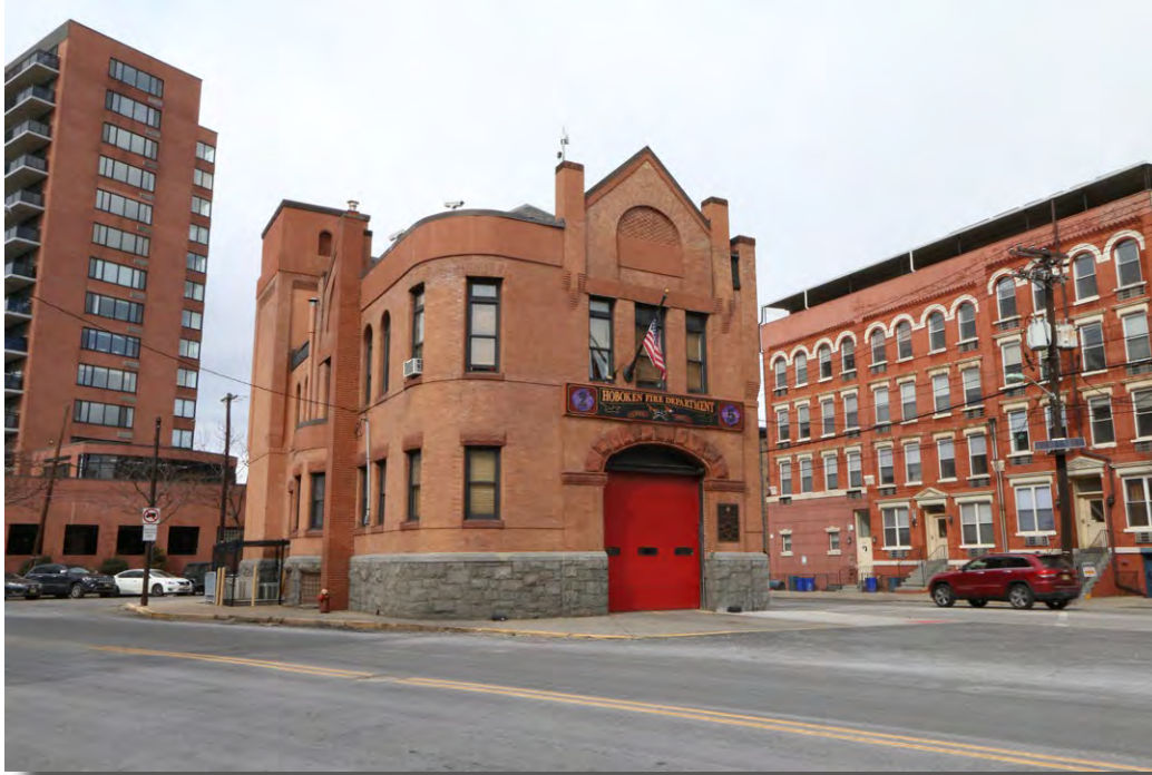
Plate 4.53: View of Engine Company #3, Truck #2 Firehouse, City of Hoboken.
