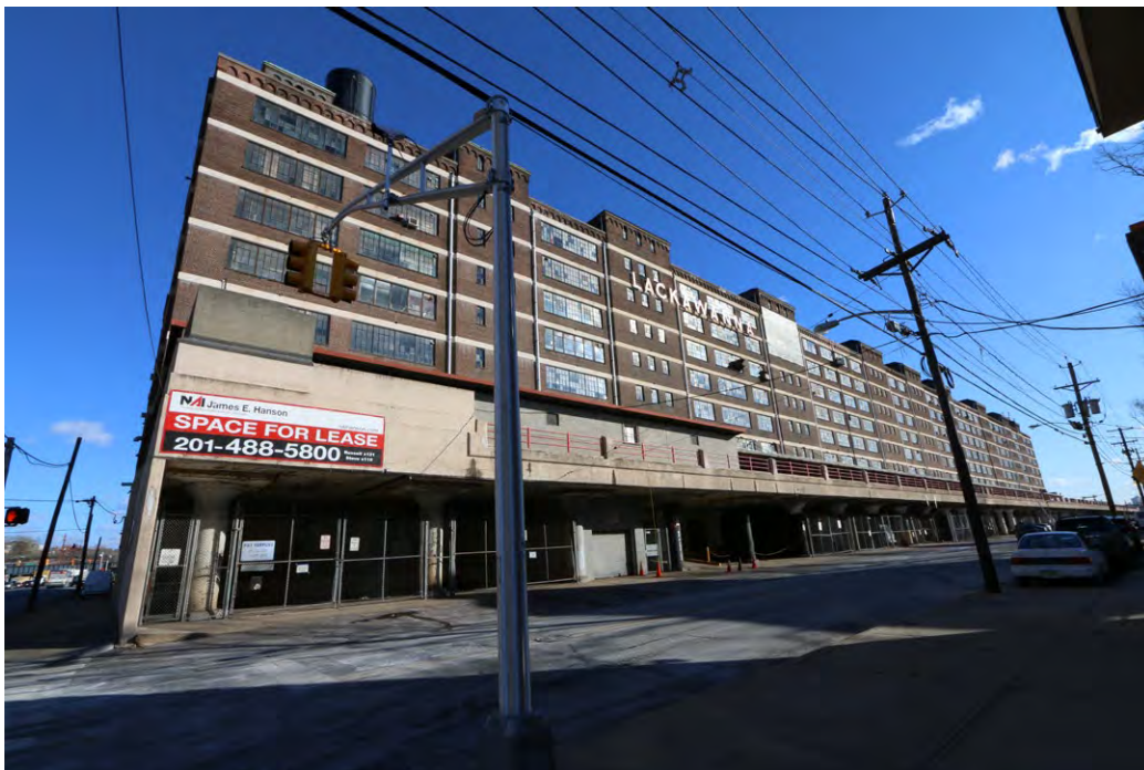
Plate 4.48: View of the Lackawanna Warehouse and Viaduct, City of Jersey City.
