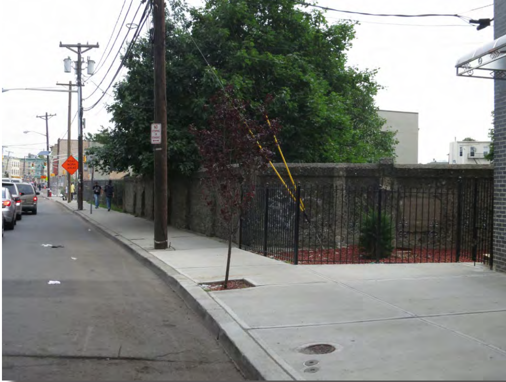
Plate 4.37: General view of the eastern wall of the Summit Avenue Bridge where it crosses the Erie Railroad Bergen Archways Historic District, City of Jersey City.
