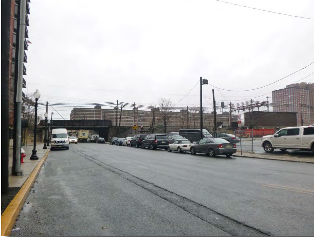
Plate 4.51: View of the Grove Street Bridge with the Lackawanna Warehouse visible in the background, on the opposite side of the Old Main DL&WRR Historic District, City of Jersey City.
