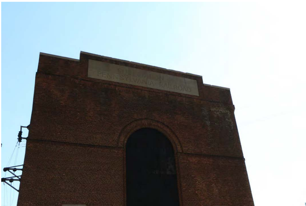
Plate 4.28: Detail of Substation 4's inscribed limestone panel on the primary elevation.
