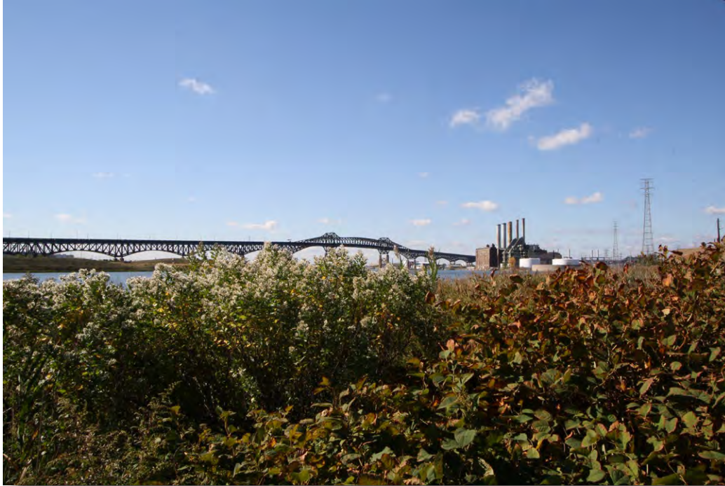
Plate 4.29: General view toward the Hackensack River, with a view of the US Route 1 Extension Historic District, the US Route 1&9 Historic District, and the PSE&G Kearny-Essex-Marion Interconnection Historic District, with the Kearny Generating Station at right, Town of Kearny.
