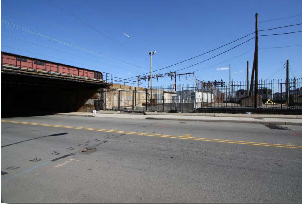
Plate 4.15: View of the Henderson Street Substation and the Old Main DL&WRR Historic District, City of Jersey City.
