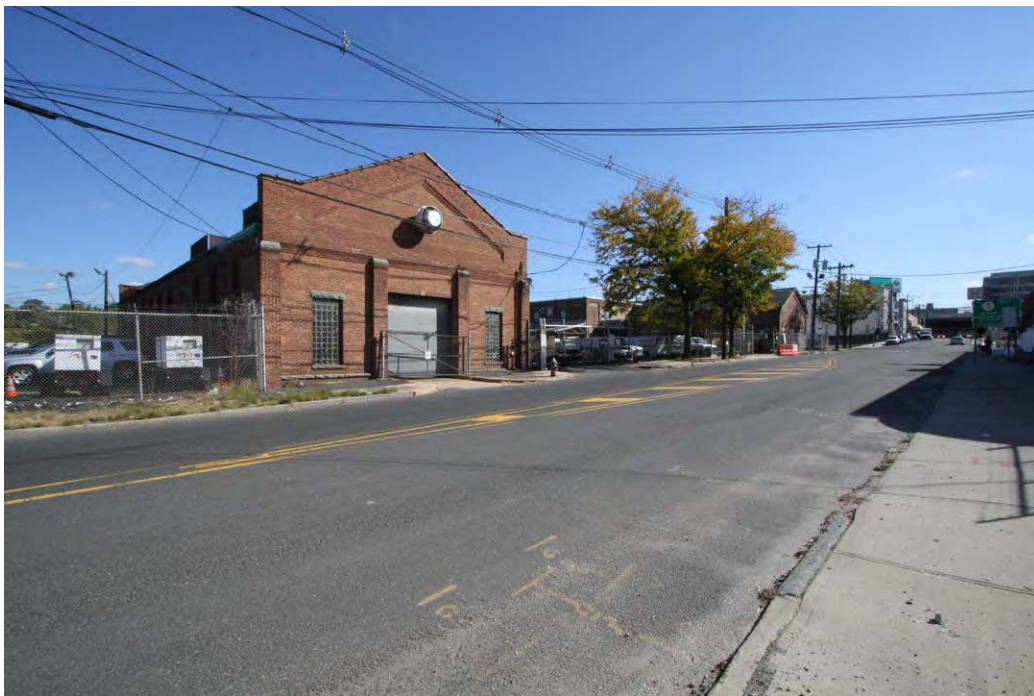
Plate 4.32: Overview, City of Jersey City, with a general view of the People's Gas Light Company/PSE&G Marion Office Historic District.
