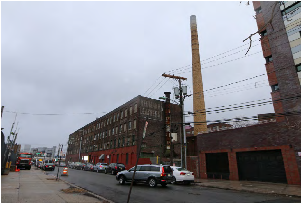
Plate 4.57: View of the R. Neumann & Co. Factory Complex toward the DL&WRR Historic District, City of Hoboken.
