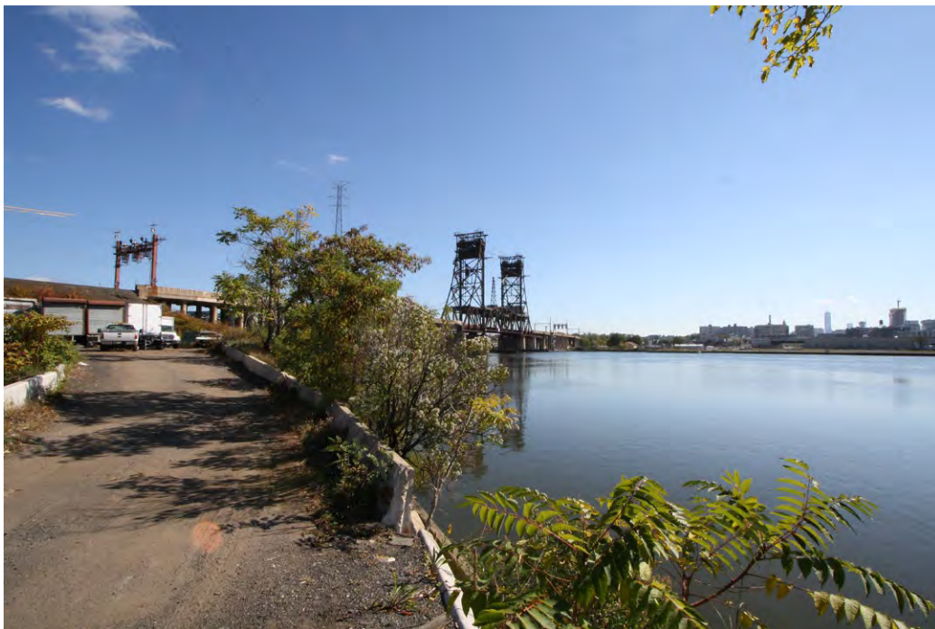
Plate 4.8: General view of the Lower Hack Draw Bridge along the Old Main DL&WRR Historic District as it crosses the Hackensack River, Town of Kearny.
