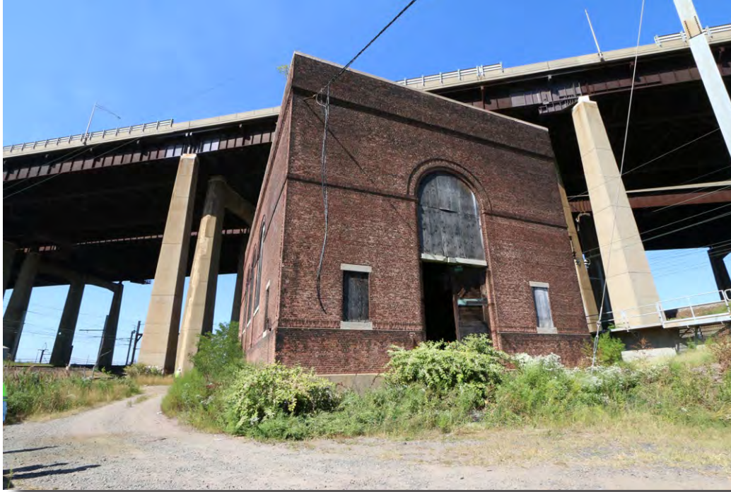
Plate 4.27: View of Substation 4, looking toward the Pennsylvania Railroad New York to Philadelphia Historic District right-of-way.
