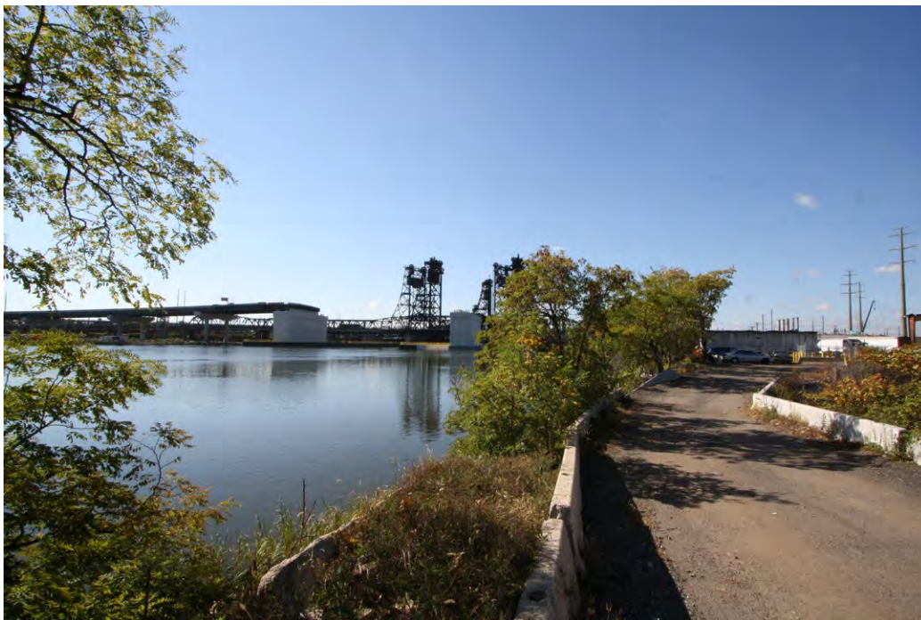
Plate 4.10: General view of the Wittpenn Bridge and the Pennsylvania Railroad Harsimus Branch (Conrail/CSX) Bridge, part of the Hackensack River Lift Bridges Historic District, over the Hackensack River, Town of Kearny.
