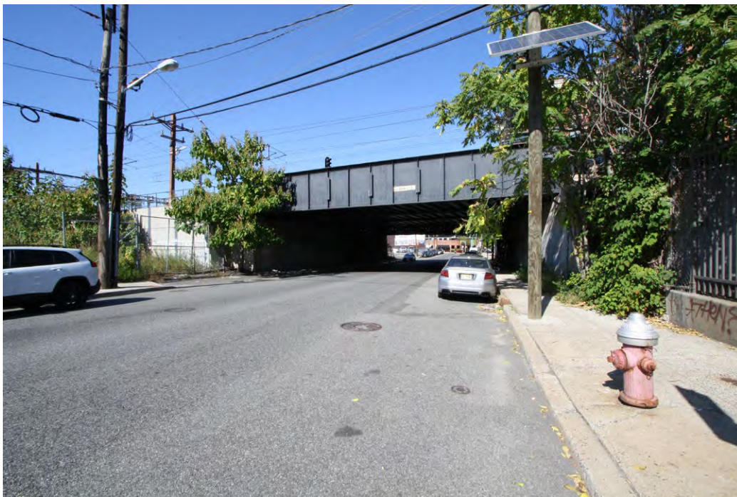
Plate 4.52: View of the Grove Street Bridge carrying the Morris & Essex line, City of Jersey City.
