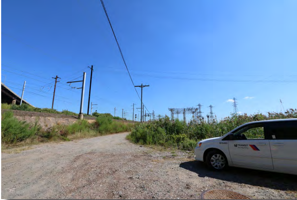
Plate 4.19: Overview, Town of Kearny, looking toward the Pennsylvania Railroad New York to Philadelphia Historic District with the Substation 41 at right.
