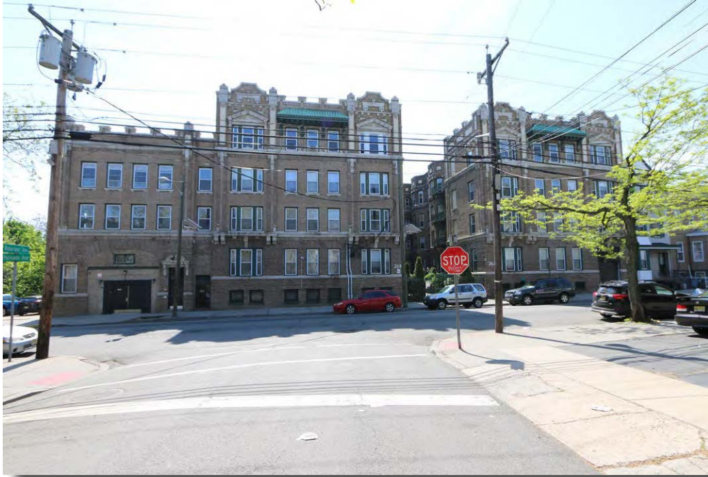
Plate 4.55: View of Belvedere Court, City of Jersey City.
