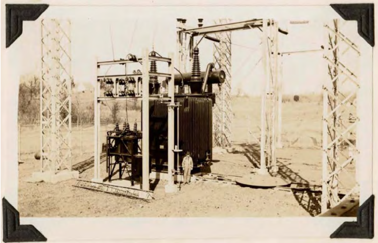
Figure 4.4: 1935 photograph of a G.E. transformer #1 with breaker in the substation in Landover, Maryland (Flagg 1935:30).
