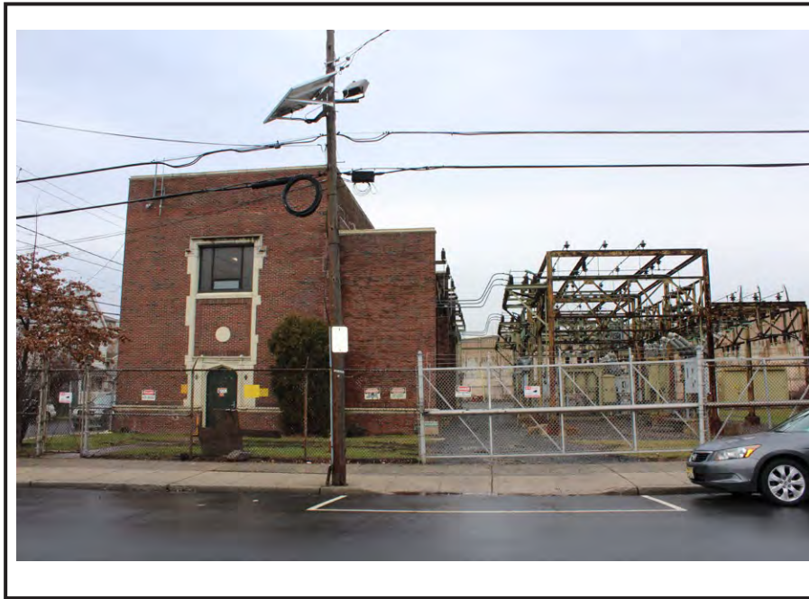
Southeast elevation of Bergen Point Substation, brick firewalls, and yard with transformers and gantries.
