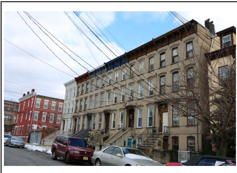
North elevation of the 252-262 Suydam Avenue.
