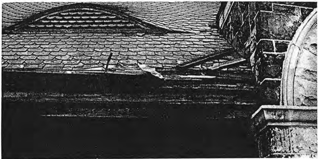
Detail of roof and front arch of West face.
