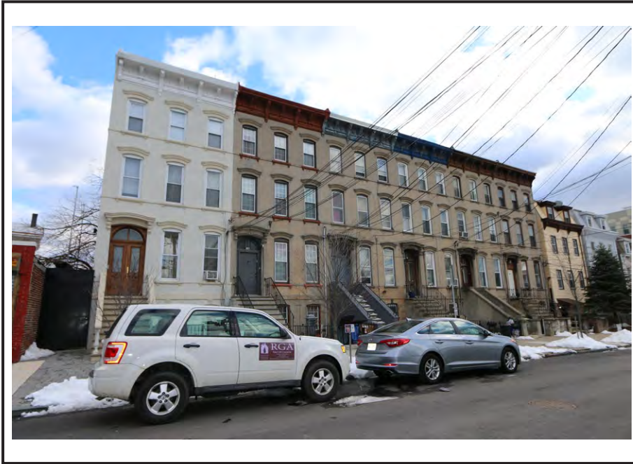
North elevation of 252-262 Suydam Avenue.
