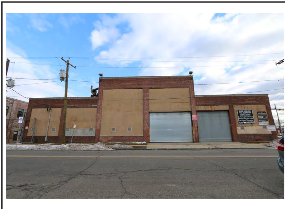
Primary Elevation view of the Westinghouse Electric Elevator Company addition.
