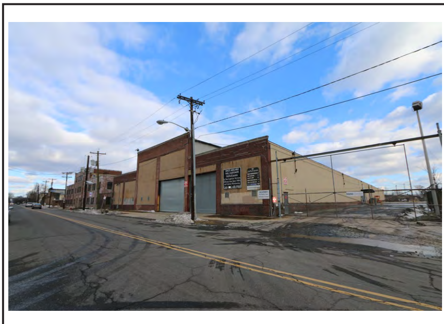
View of all three buildings with the Westinghouse Electric Elevator Company addition in the foreground.
