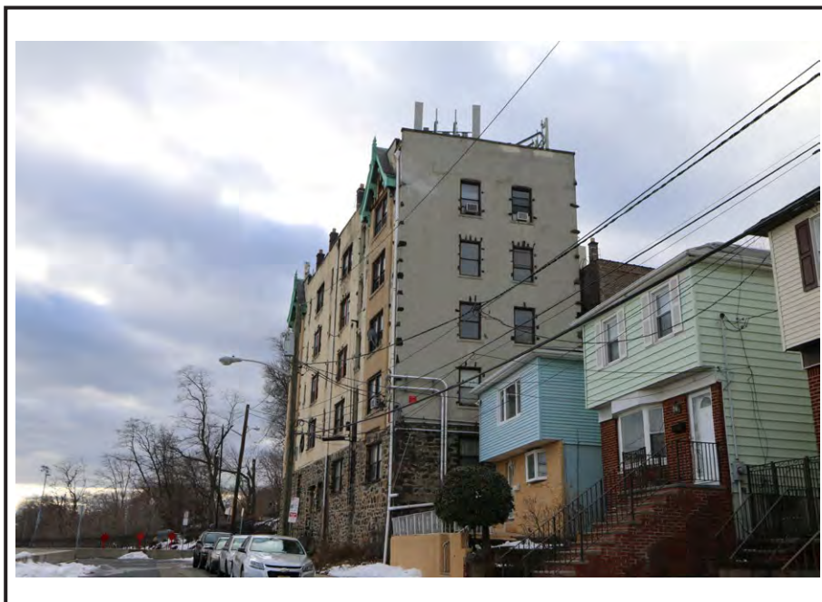
The partial view of the east elevation.
