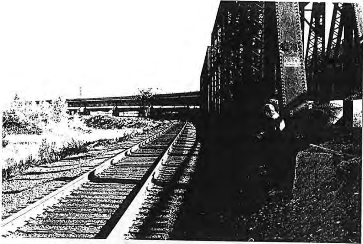
2. Conrail Bridge 2.77 Facing Northeast January 1994
