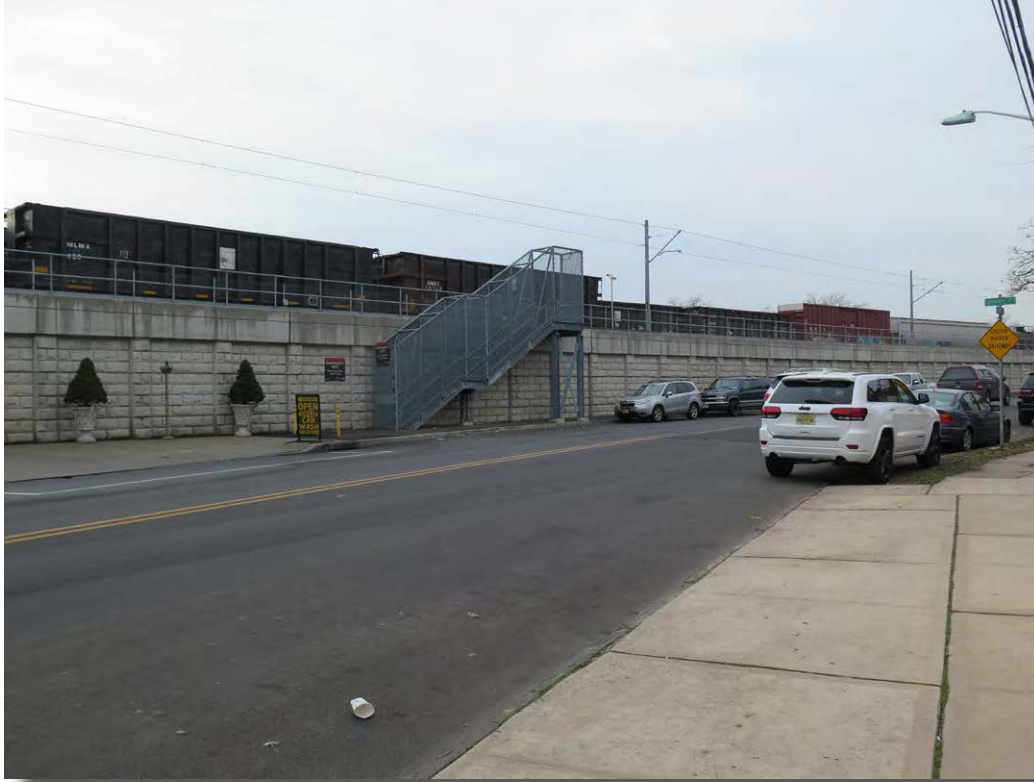
Plate 5.7: View of HBLR from the intersection of Avenue E and East 14th Street, City of Bayonne. Taken from the approximate location of Site 28-Hd-1.
