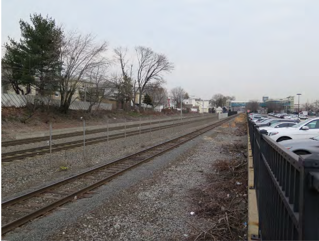
Plate 5.9: Overview of HBLR tracks at Thirty-fourth Street Station, City of Bayonne.
