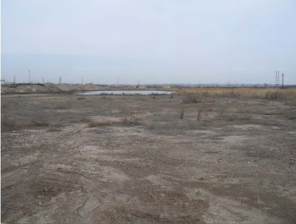
Plate 5.3: Overview of Main Facility Electric Yard.
