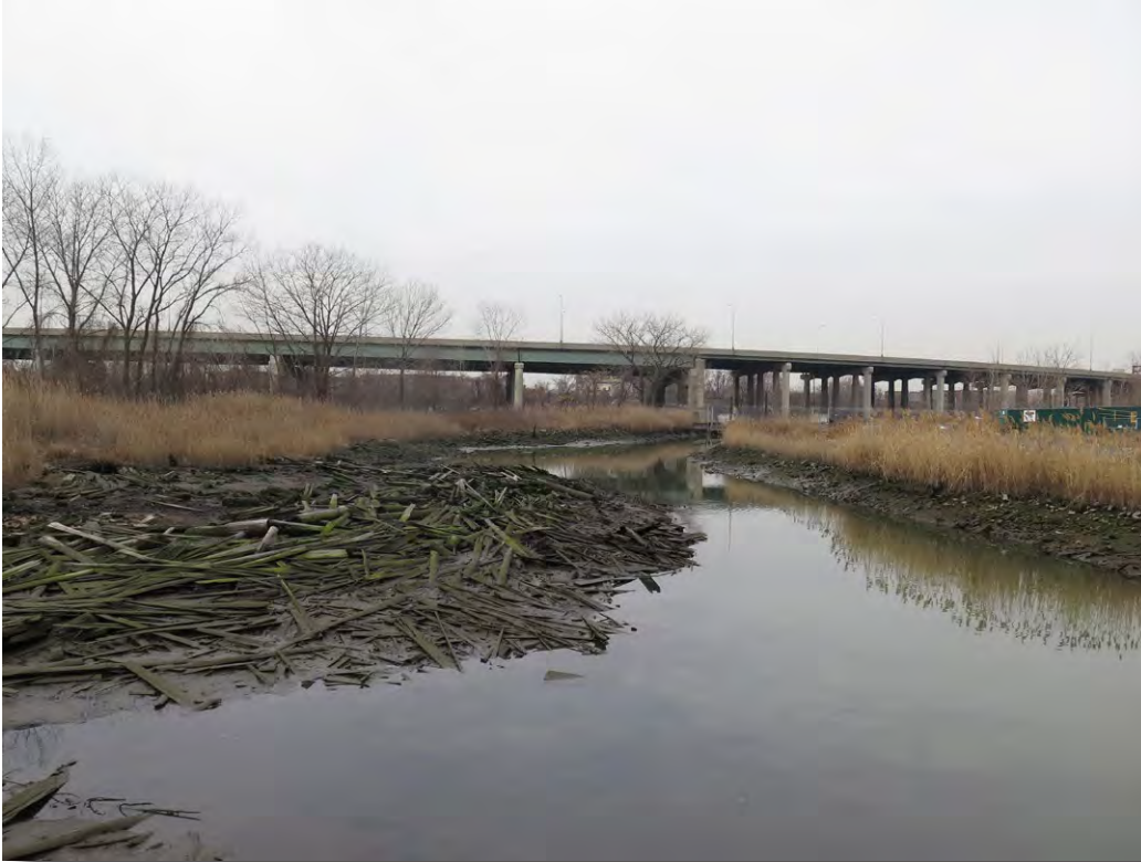
Plate 5.21: View toward HBLR and Interstate 78 from the approximate location of Site 28-Hd-52, City of Jersey City.
