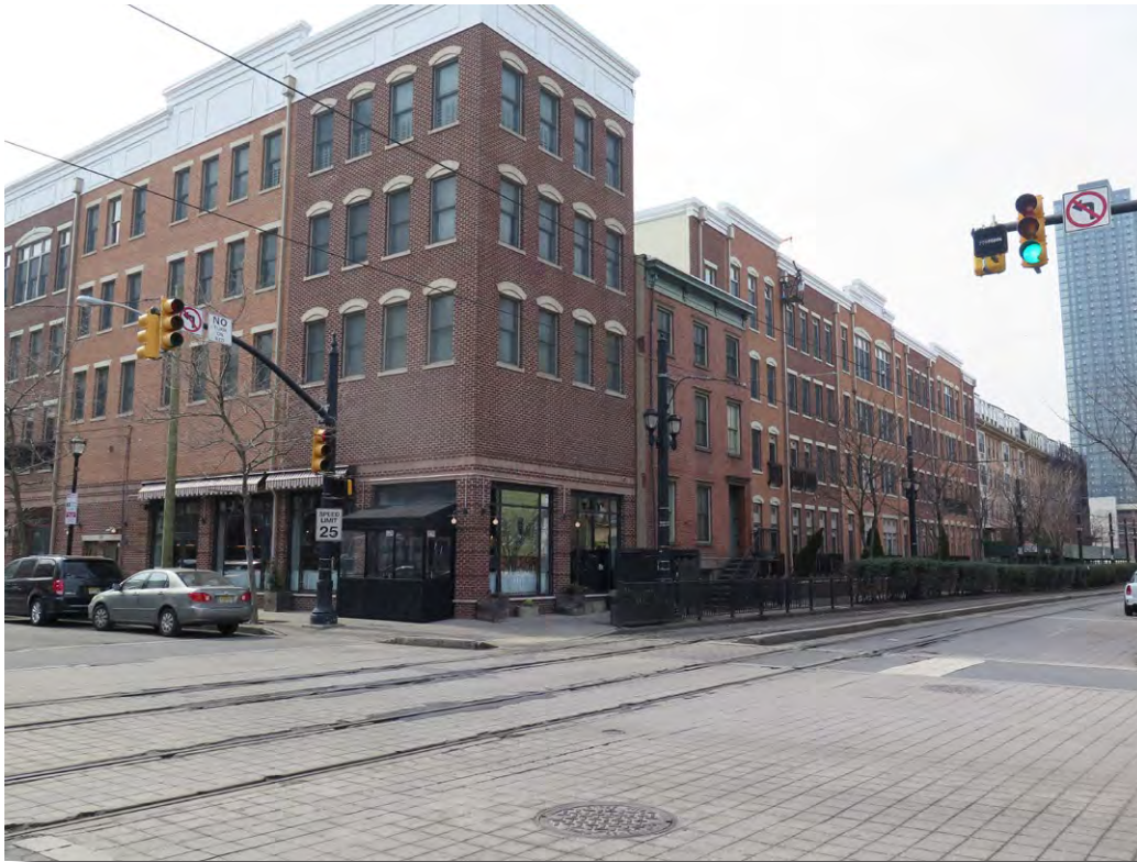
Plate 5.23: Existing conditions at approximate location of Site 28-Hd-53, Corner of Warren Street and Essex Street, City of Jersey City.
