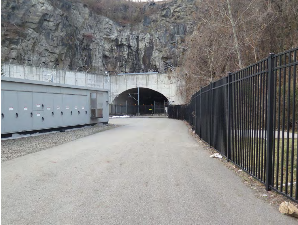
Plate 5.29: View of eastern end to the HBLR's West Shore Tunnel.
