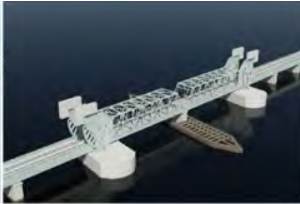
Bascule Span
