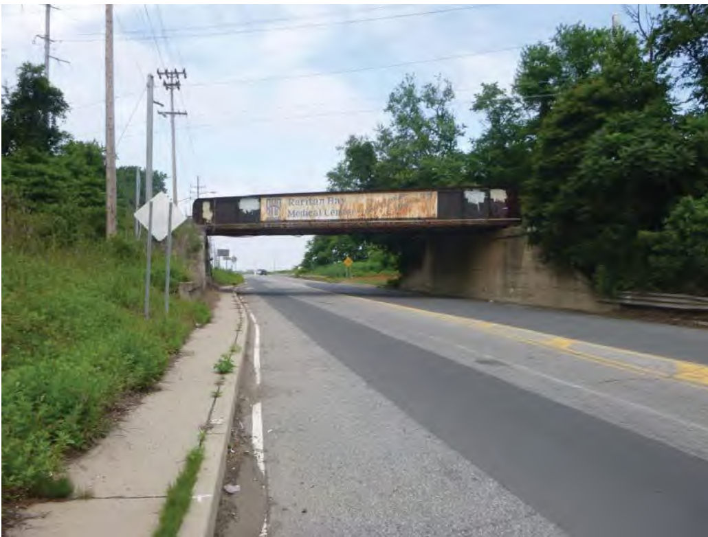
Plate 14: Overview, through Plate Girder Bridge (No. 60.71) Carrying PRR Interchange Track over Main Street, South Amboy.
