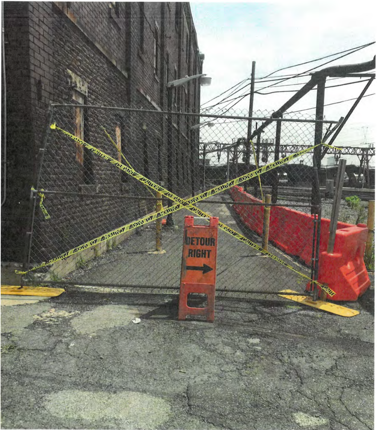
The area along the south side of the building was already secured with barricades against falling bricks. As noted in the photos below the south parapet has failed presenting a hazard to workers who normally traverse this area.
