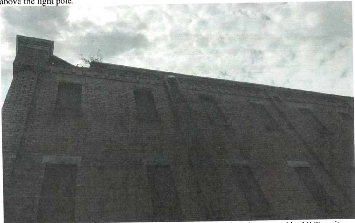
At the north wall the parapet has failed and was being removed on the east end by NJ Transit forces at the time of the inspection.
