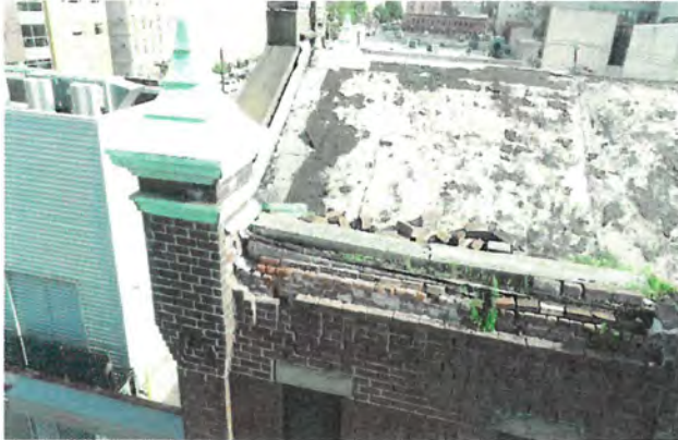
Photo 3: Diagonal crack below the cornice
