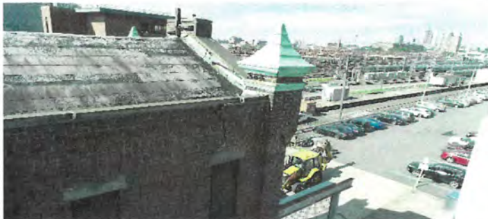
Photo 5: Separation of cornice at a different location
