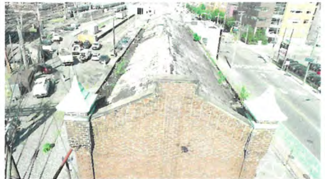
Photo 4: One of the cornices separated by crack from the adjacent brick wall
