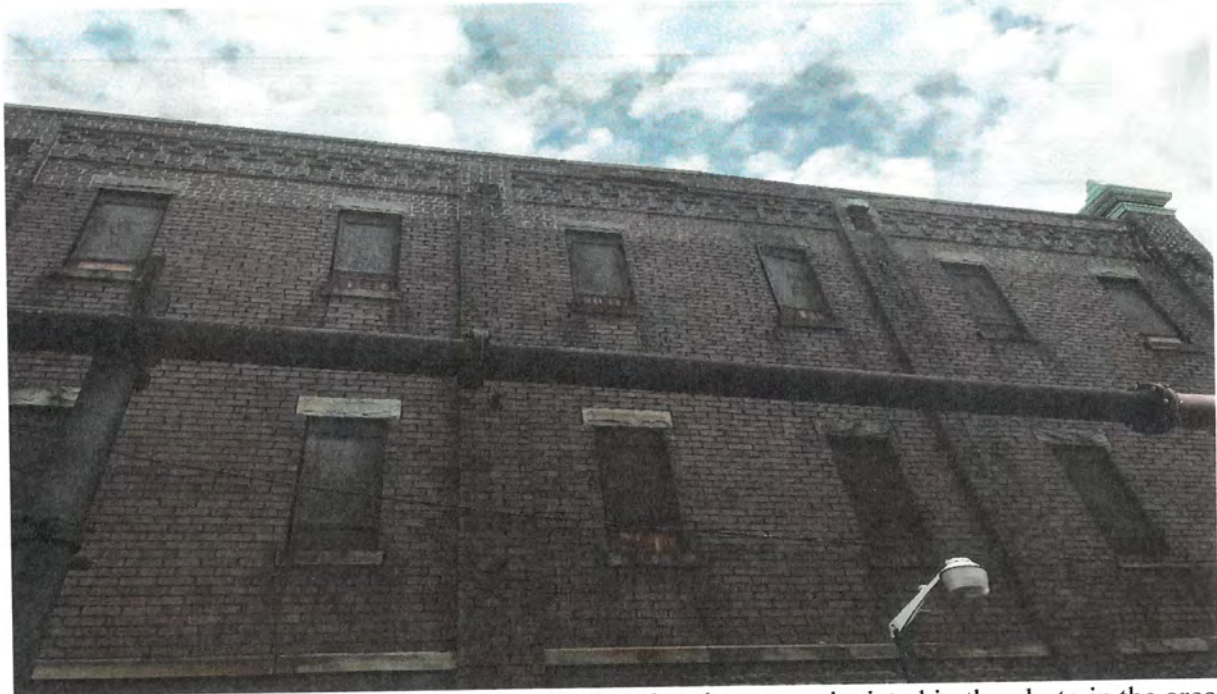
The parapet along the south wall was also displaced at the top as depicted in the photo in the area above the light pole.
